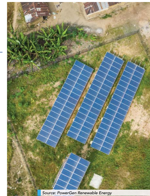
Source: PowerGen Renewable Energy
